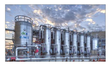
Cambi's Thermal Hydrolysis Process (CambiTHP®) is a proven and reliable technology for treating wet organic waste (sewage sludge, biowaste etc.) It enhances the anaerobic digestion and biogas production. Since 1992, Cambi has developed approximately 60 projects in 20 countries, being at the forefront of the global market for thermal hydrolysis and sustainable sludge manage-
